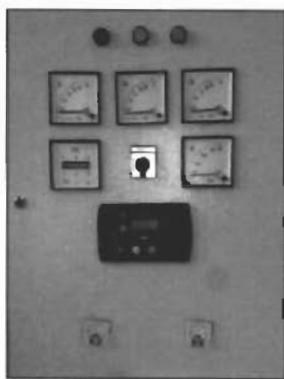
AMF (*Automatic Mains Failure*)
